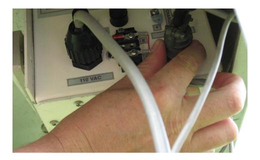
3. Remove the clutch arm bolt and associated hardware from the push rod and motorbox. The push rod will swing free. Save the bolt, washers (2, bronze and nylon), and the bronze bushing to re-use when installing the replacement motorbox.
